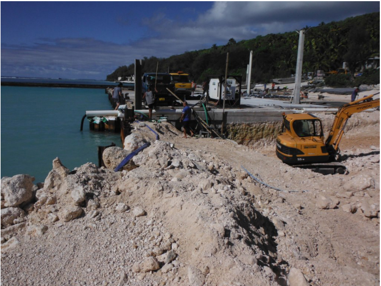
Figure 6. The harbour construction under way (photo taken on 10 February 2014).
